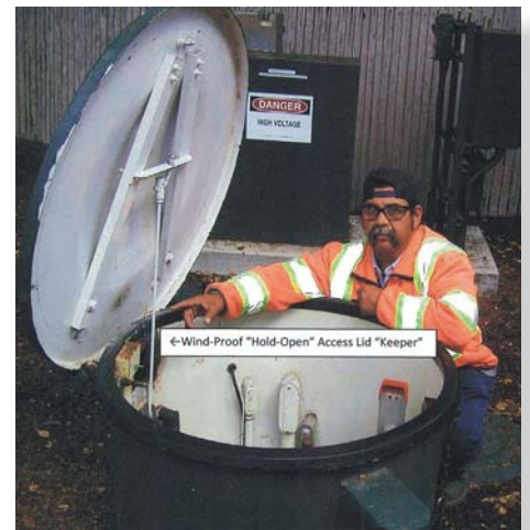
Juan Moreno, Maintenance Technician II, from Pebble Beach Community Services District, displays the "lid-keepers" he designed.
