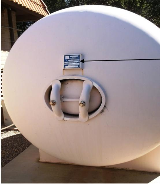
All metal vessels used as hydropneumatic or surge tanks must be constructed to American Society of Mechanical Engineers (ASME) standards or be Code-certified. This can often be verified by reviewing the manufacturer's plate installed at the time of construction.
