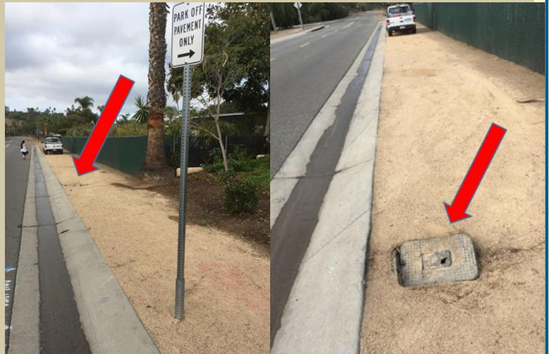
Meter boxes may be installed in areas subject to traffic. In most cases, these areas are known at the time of installation and the appropriate type of meter box and lid is installed by the utility. In other cases, due to development, the type of meter box may change.
