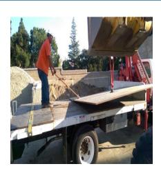
**Problem:** Difficult to safely maneuver and position heavy road plates being hoisted into or out of position. Plates are guided into position with a square shovel requiring employees to stand too close to the plate.
