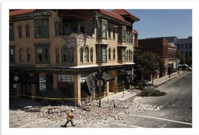
Napa earthquake 2014—magnitude 6.0
