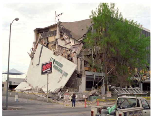
Northridge earthquake Kaiser Permanente Building collapse 1994—magnitude 6.7
