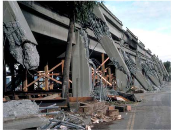
Loma Prieta earthquake damage in Oakland 1989—magnitude 6.9
