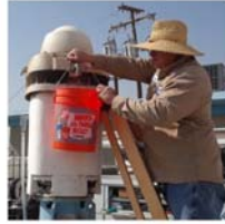
Filling the electric motors with oil
