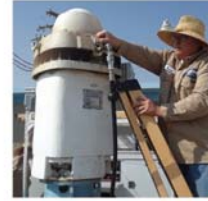
Filling the electric motors with oil
