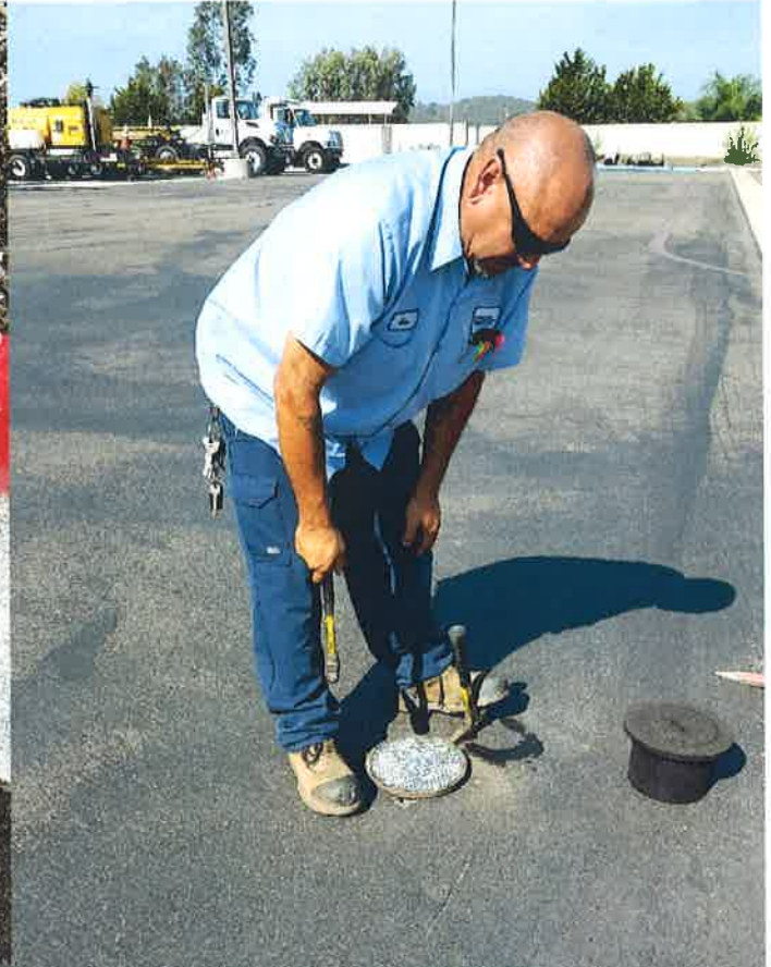
Traditional valve lid removal method – non slotted
