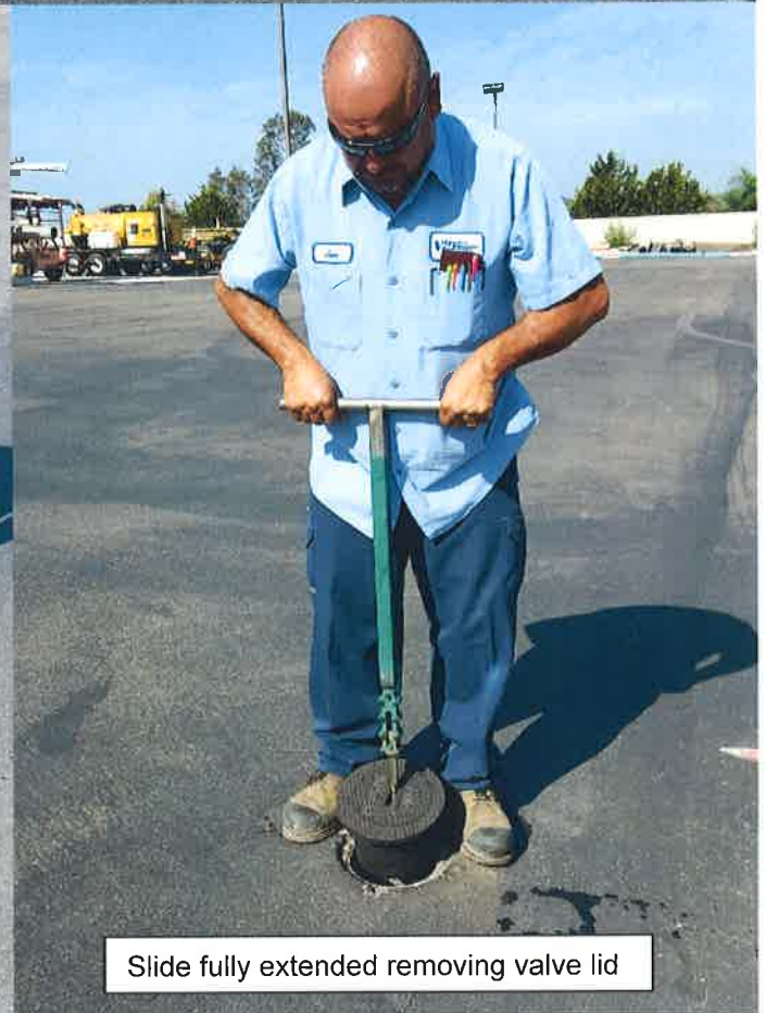
Traditional valve lid removal method – non slotted
