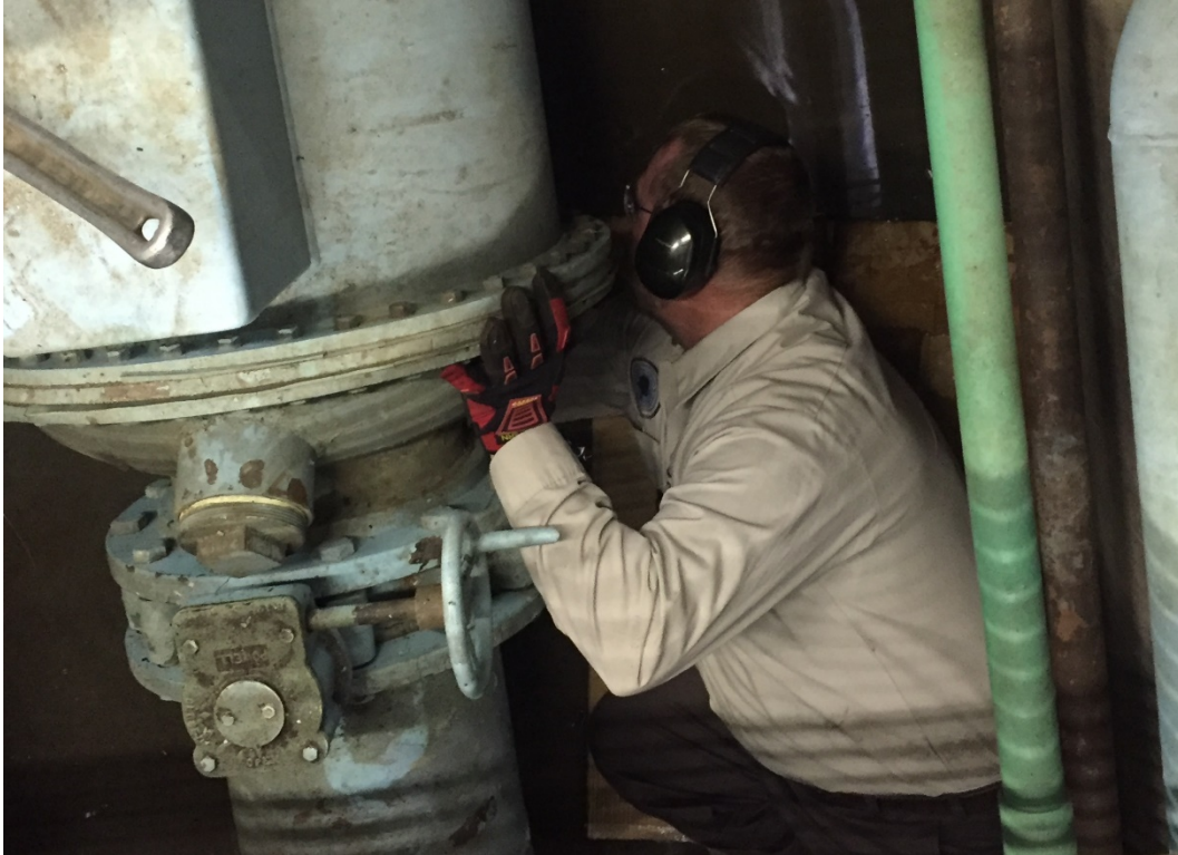
FIGURE 5 – MECHANIC REMOVING PLUG AT LOWER HAND HOLE
