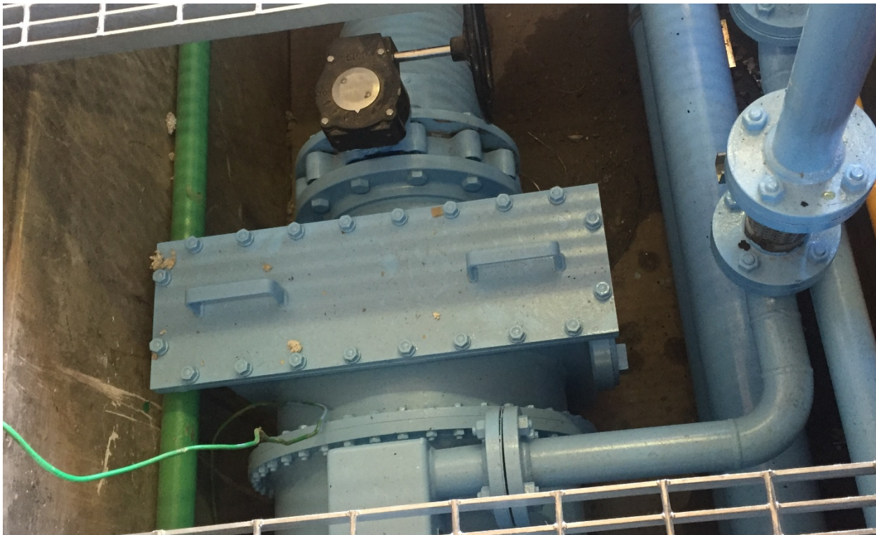
FIGURE 8 – NEW FILTER BOX SCREEN ASSEMBLY (IN PLACE)
