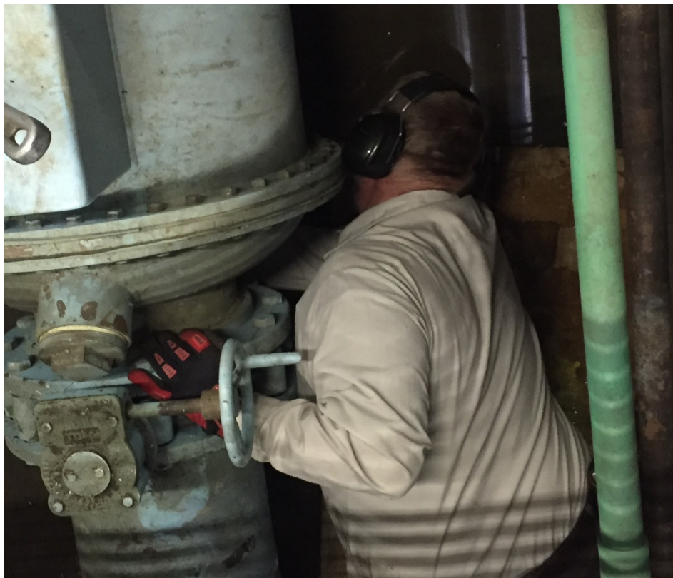
FIGURE 6 – MECHANIC ACCESSING LOWER HAND HOLE
