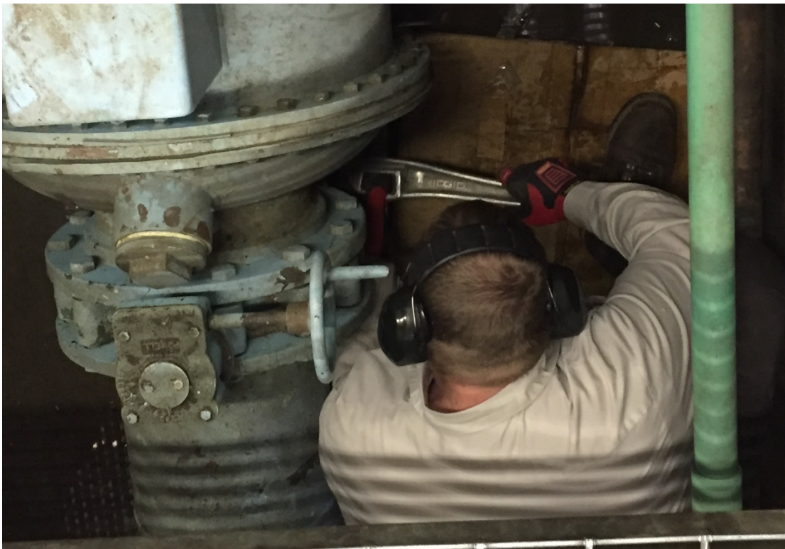
FIGURE 4 – MECHANIC REMOVING HAND HOLE PLUG (IN WELL BELOW FLOOR)
