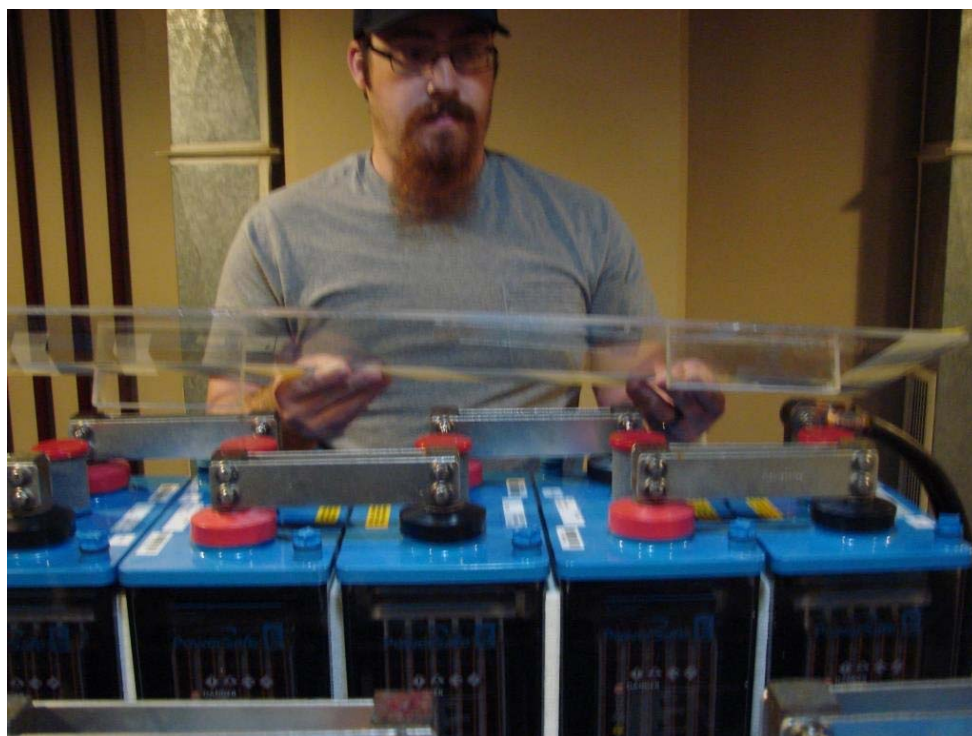
Securing battery cover into place
