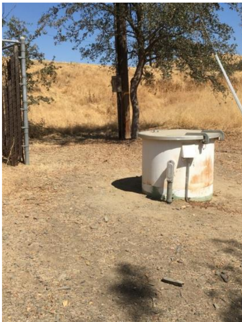
Old Lift Station
