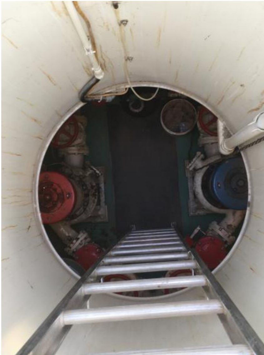
Old Lift Station
