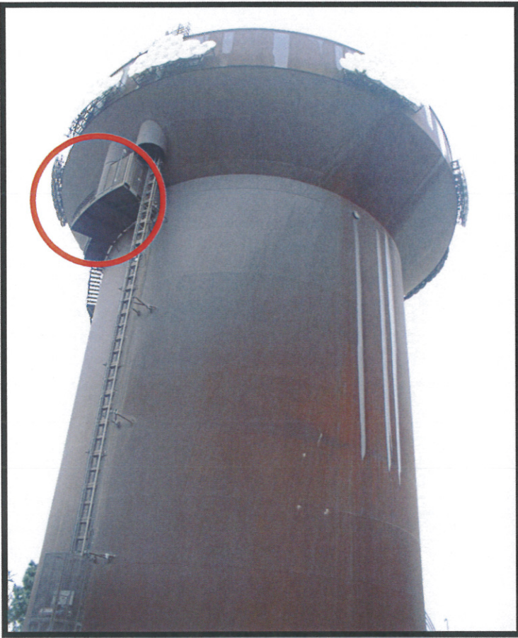
Tank landing with guardrail - approx. 100 feet up
