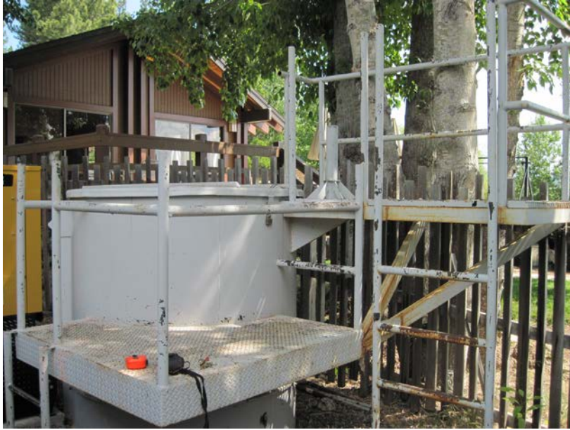
Park Terrace Sewer Station Before
