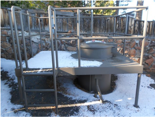
Water's Edge Sewer Station – After
