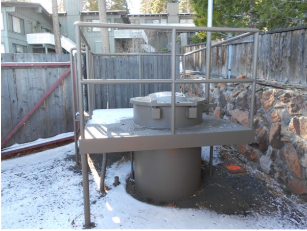
Water's Edge Sewer Station - After
