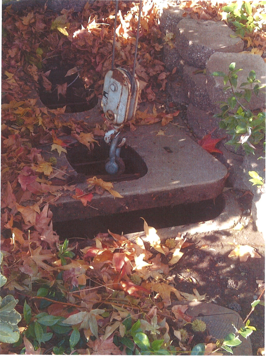
Meter box lid being lifted by crane using lifting apparatus.
