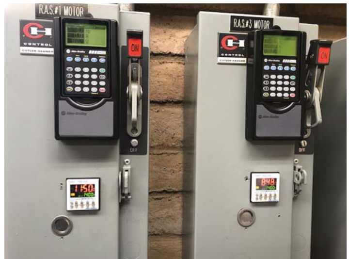
Ramona MWD installed external controls on the outside of the electrical cabinet along with a digital timer for pumping time control at their Wastewater Treatment Plant.
