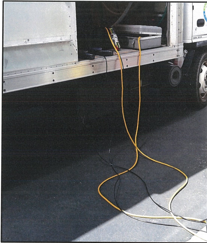
Before: Electrical Cord Trip Hazard
