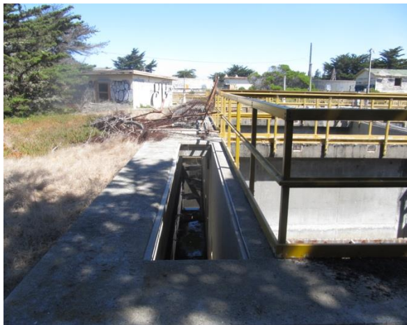
Photos 3 & 4 – Abandoned Old Ord Plant facilities including unsecured access to confined spaces and vandalism
