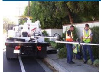
Similar to the handheld powered or hydraulic valve turning tools, vehicle-mounted equipment eliminates the repetitive motion of turning the valve. Additionally, the torque required to operate the valve is transferred to the vehicle and not the operator.
