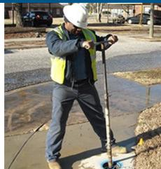
The operator adjusts the length of the tool to place the handle within their "power zone." The "power zone" is defined as the space between the shoulder and the waist, providing the greatest strength and balance. Manual tools, however, do not eliminate the potential torque or repetitive movement the operator may experience. Fortunately, districts can further reduce risks by adopting an administrative control practice were two operators alternate turning the valve
