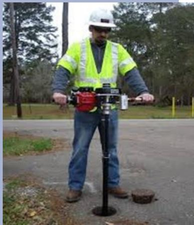
**Figure 2. Valve Operation with the Valve Boss**
