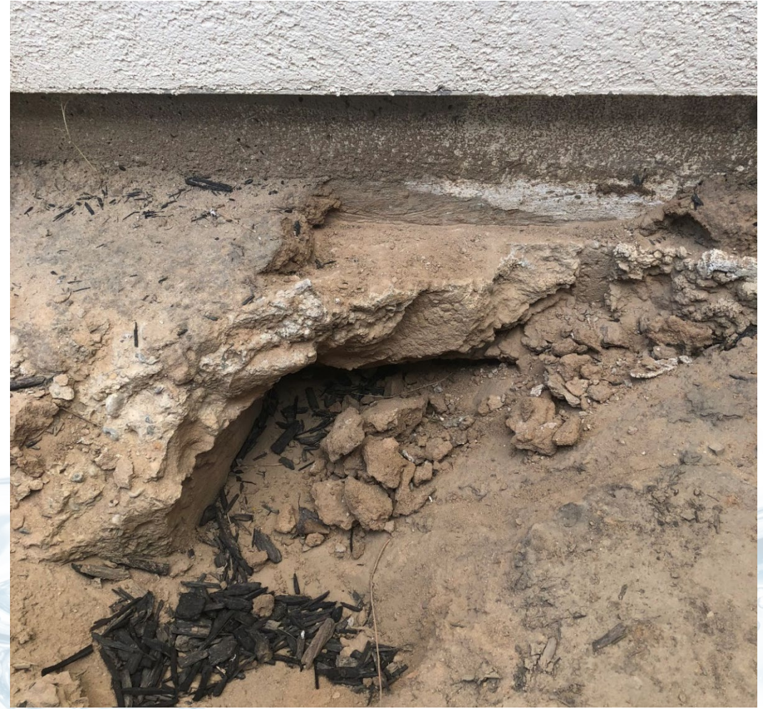
Cracked flooring due to foundation movement
