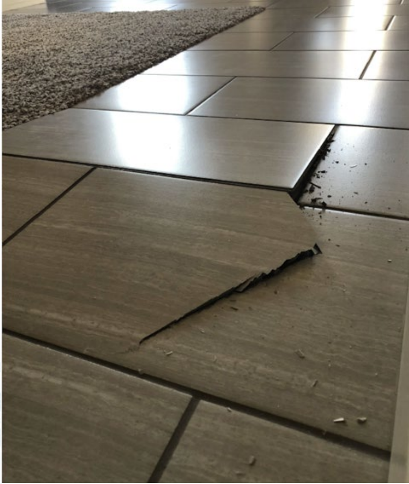
Cracked flooring due to foundation movement
