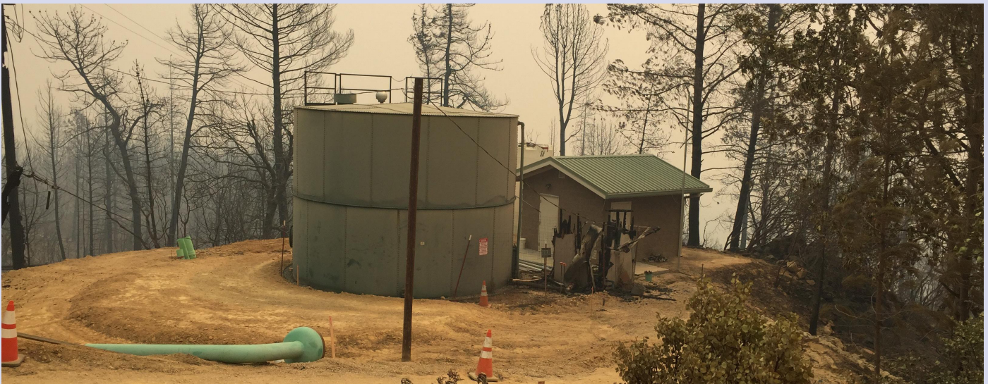
Source: PACE Engineering, Shasta CSD Upper Brunswick Pump Station alongside remains of the old wood frame pump station after the fire.
