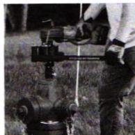
Valve exercising is the process of manually or automatically opening and closing valves to ensure they continue to function
