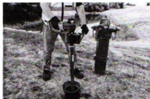
The AWWA (American Water Works Association) defines the practice of valve exercising as; "[valves] should be operated through a full cycle and returned to its normal position on a schedule that is designed to prevent a buildup of tuberculation or other deposits that could render the valve inoperable or prevent a tight shut-off."
