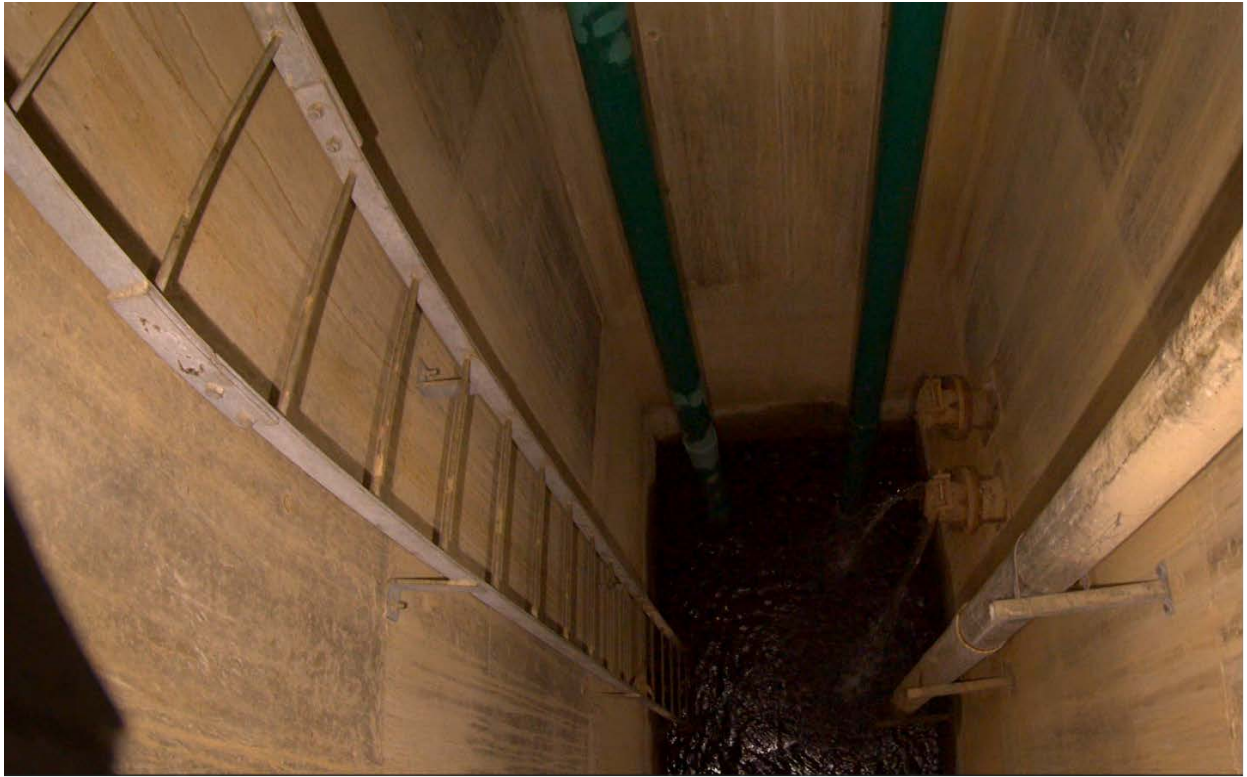
Photo 3: Drainage sump (confined space) with standing water. Access is via a vertical ladder.
