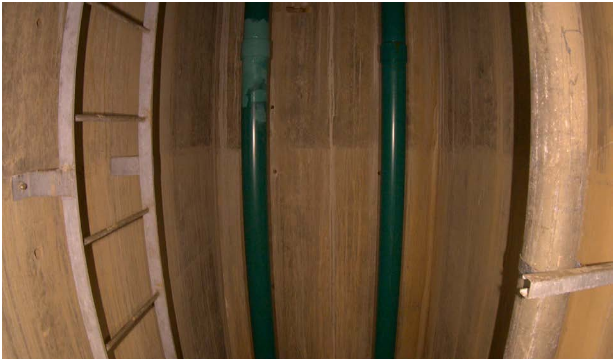
Photo 4: Drone image provides interior condition of the drainage sump
