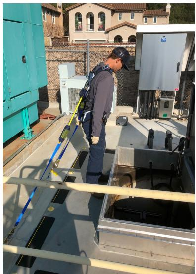
Twin Leg Lanyard is connected to temporary anchors, providing fall protection for employee when working around open Wet Well.
