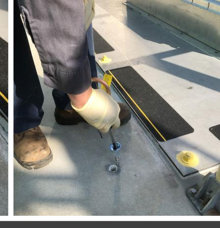
Holes were drilled into concrete (according to specs) at the face of the Wet Well, where the DBI Sala Temporary Concrete Anchors can be inserted and used as anchor points when needed. When job is complete, anchors are removed and stored.
