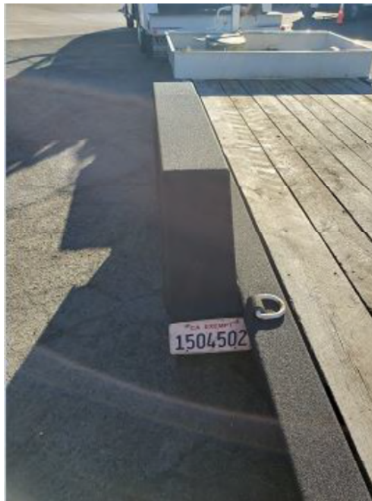
After Coating Walking/Working Surface Rhino Liner – Prevents Slipping Hazard.
